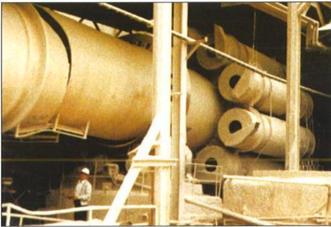
Figure 3. Catastrophic kiln shell failure.
