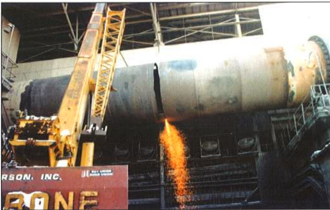
Figure 4. Removing an existing shell section.
