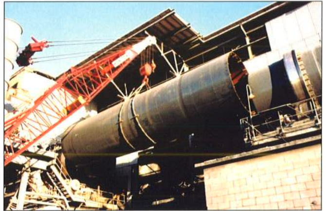
Figure 5. Installing new shell section.
